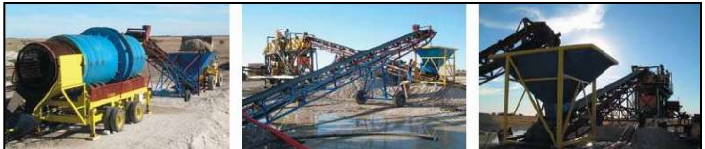
Commissioning of Bakerville plant
