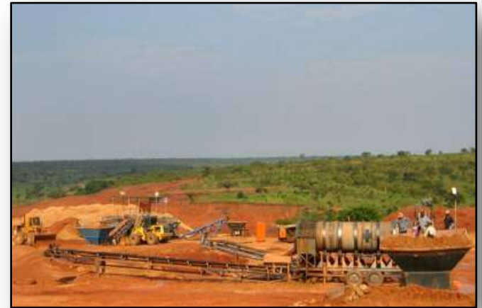
General overview of the Cassanguidi plant
