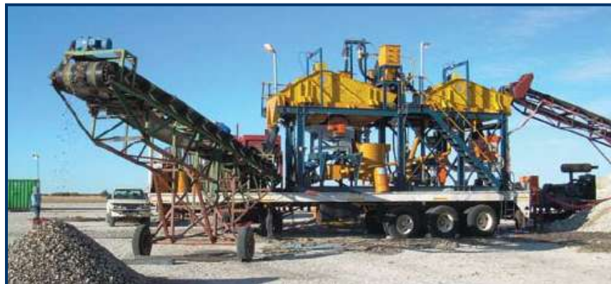
Commissioning of the Dense Medium Separation (DMS) plant, Bakerville Project
