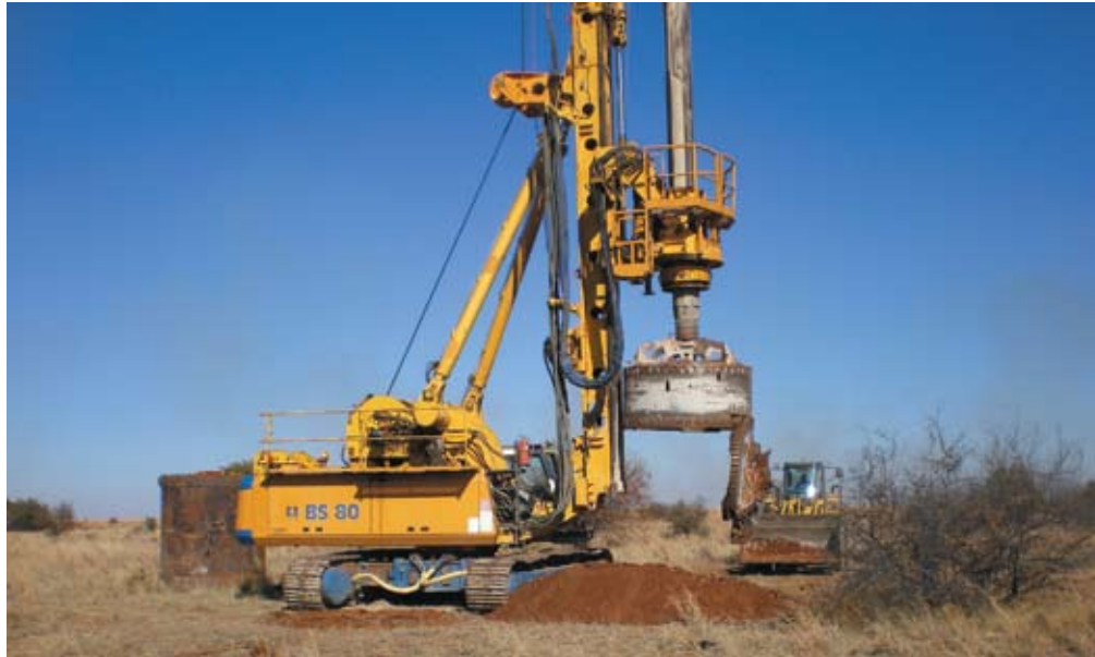
Patsema Bauer rig large diameter drilling, Patsema.
