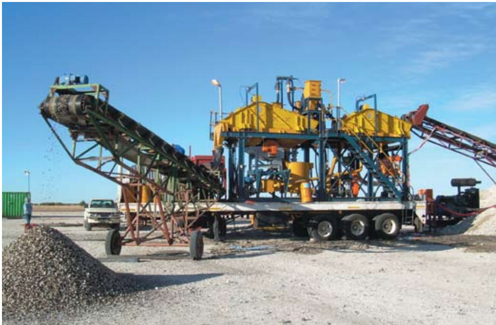
Commissioning of the Dense Medium Separation (DMS) plant, Bakerville plant.
